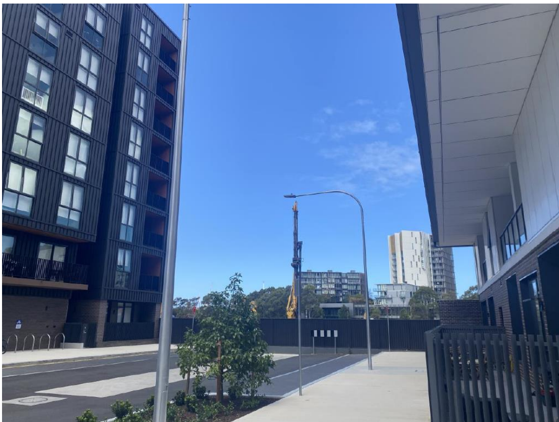
Figure 5: Site viewed from Peters Street looking east
