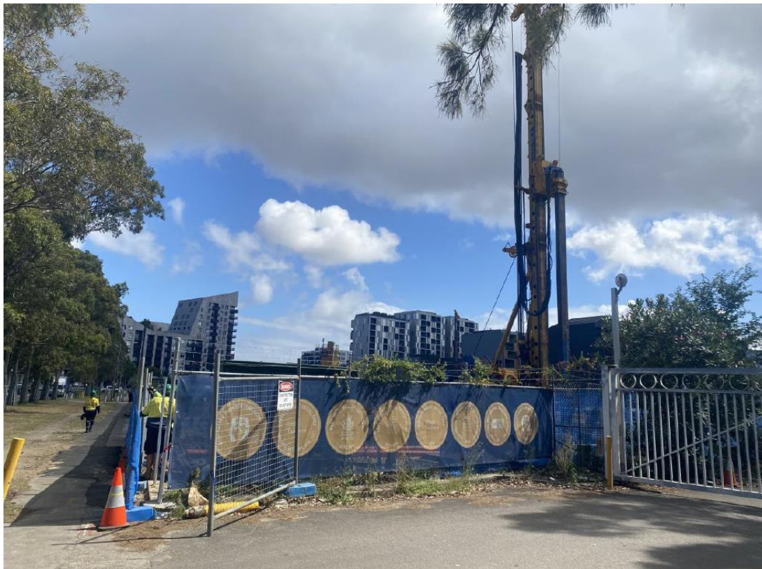
Figure 3: Site viewed from Link Road looking south
